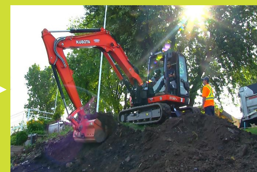
▲ Excavator in action © Denys Lortie
