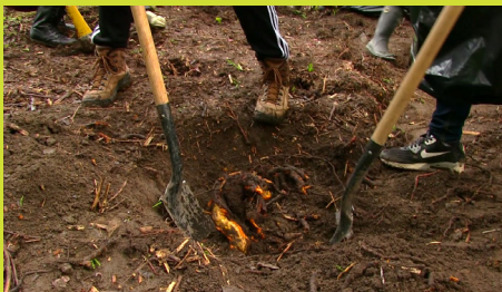
▲ Manual excavation © Denys Lortie
