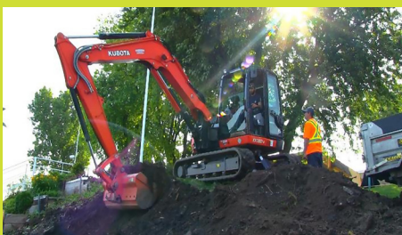
▲ Mechanical excavation © Denys Lortie
