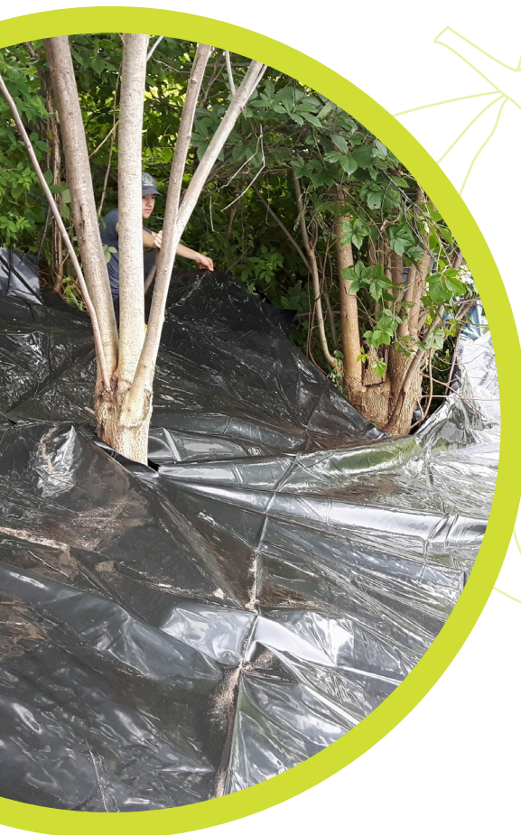
▲ Installed geomembrane © Comité ZIP Jacques-Cartier
