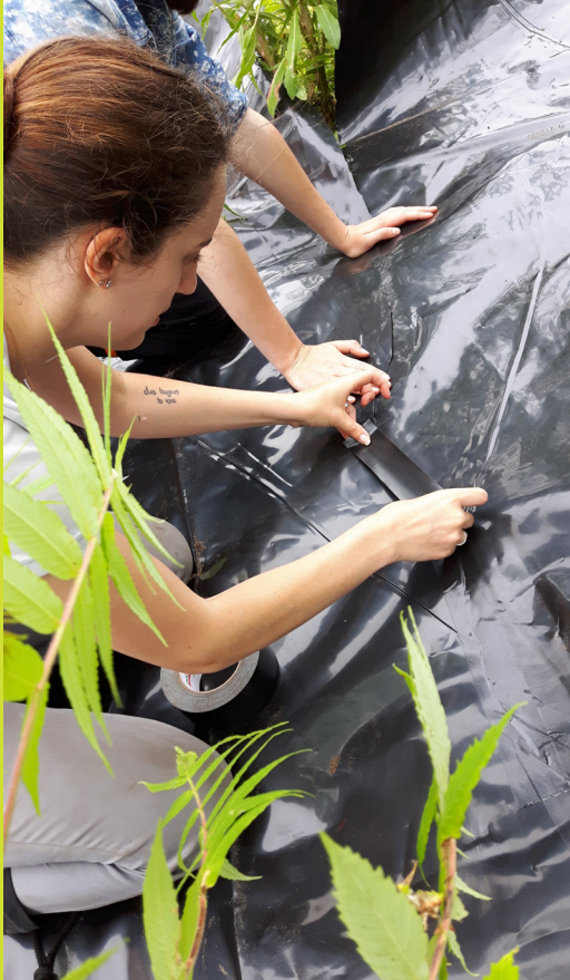
▲ Repairing a geomembrane © Comité ZIP Jacques-Cartier
