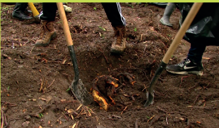
▲ Excavation manuelle © Denys Lortie
