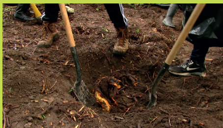
▲ Excavation manuelle © Denys Lortie
